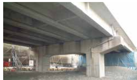
Photo-3 T-girder bridge with the electrochemical desalination ▶
