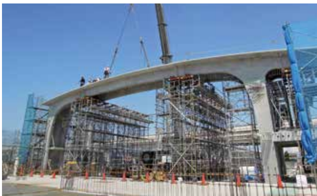
Photo-2 Erection of roof beams
