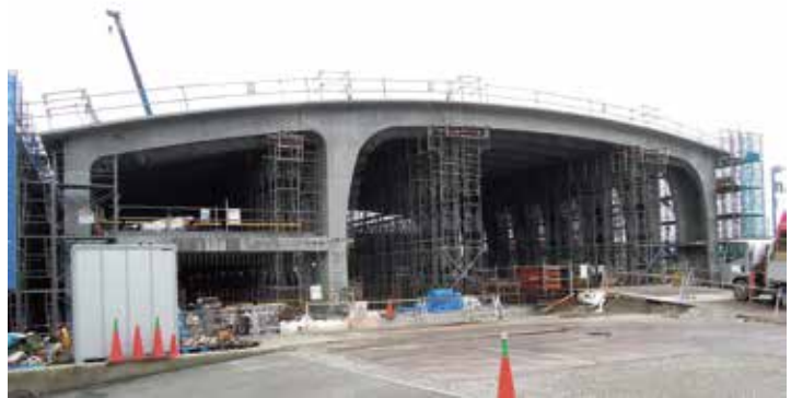
Photo-1 Completion of precast members assembly
