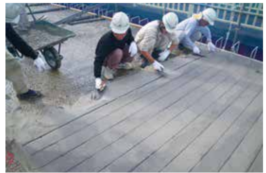
Photo-3 Erection of resin mortar and CFPR rod
