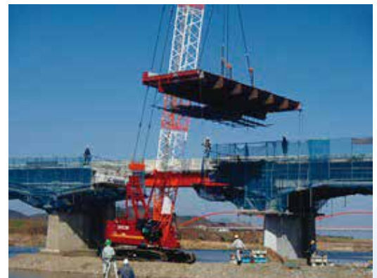
Photo-4 Steel bridge erection status
