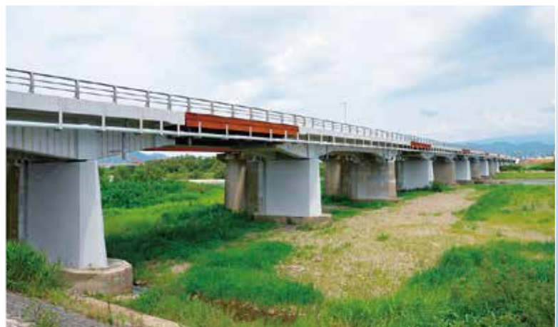
Photo-1 Renewal and reinforcement works completed
