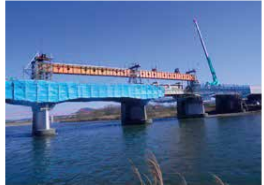
Photo-2 Removal of suspended girders using erection girders
